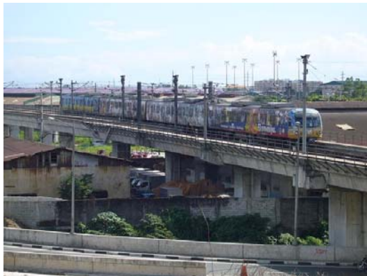
Line 2 train running near Santolan Station
